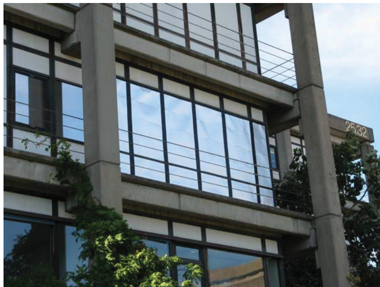
Figure 10.4 Photograph of the reflector coated insulation material covering the south side wall of the laboratory.
