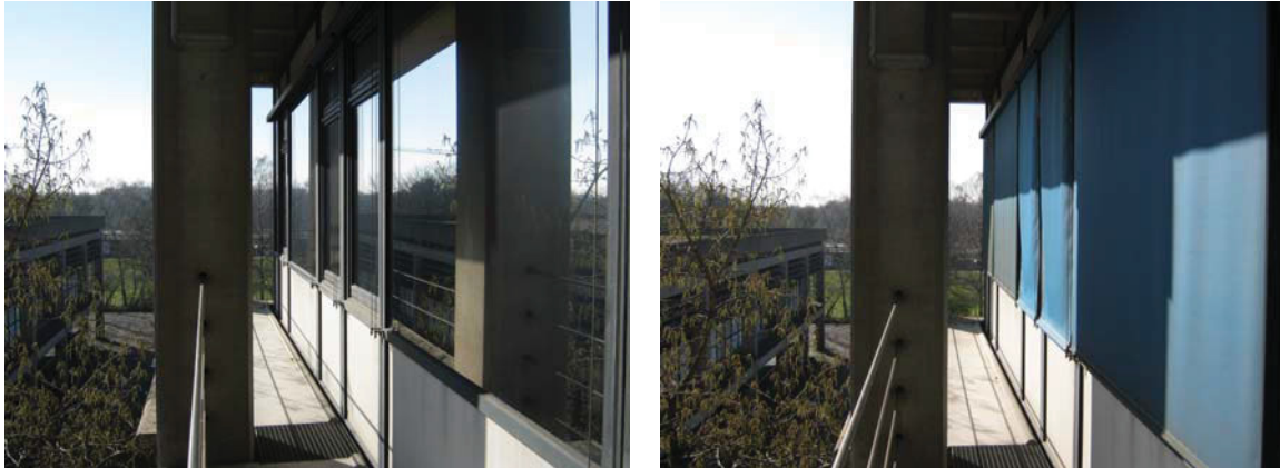
Figure 10.3 Photographs of the reflective tint window film covered windows (left) and the roller aprons (right) used for reduction of the sun irradiation.
