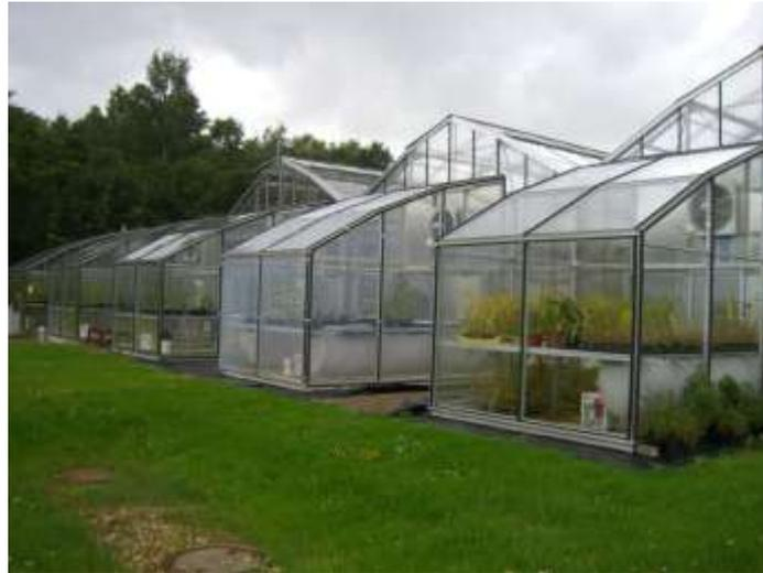
**Figure: 1** Greenhouses at Forschungszentrum Jülich covered with cladding materials differing in transmittance of UV-B. The Float glass (control glass, first glass from the right) passes nearly no UV-B radiation, MMAR glass (a multistructured glass, the second glass from the left) is the “intermediate” treatment concerning UV-B transmittance, whereas newly developed ETFE foil (the second on the right) showed high UV-B transmittance.
